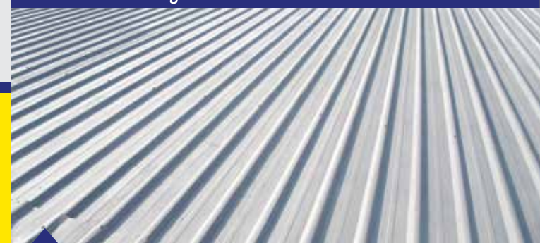
Atap Asbes & Atap Metal
