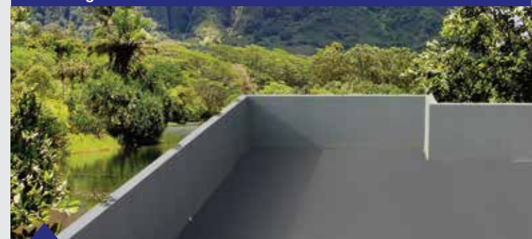
Dak Beton & Talang Beton
