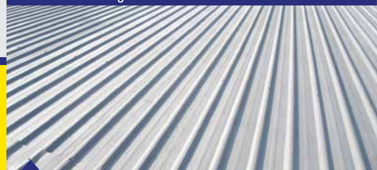
Atap Asbes & Atap Metal
